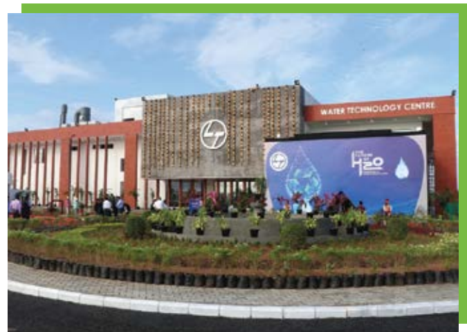
L&T Water Technology @Kanchipuram
