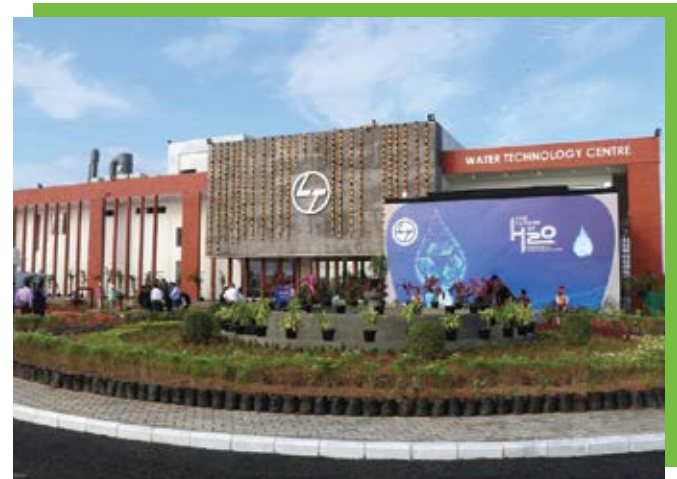
L&T Water Technology @Kanchipuram
