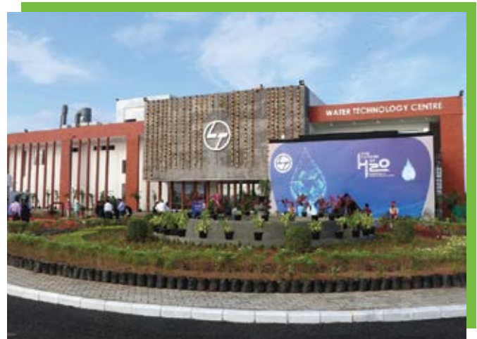
L&T Water Technology @Kanchipuram
